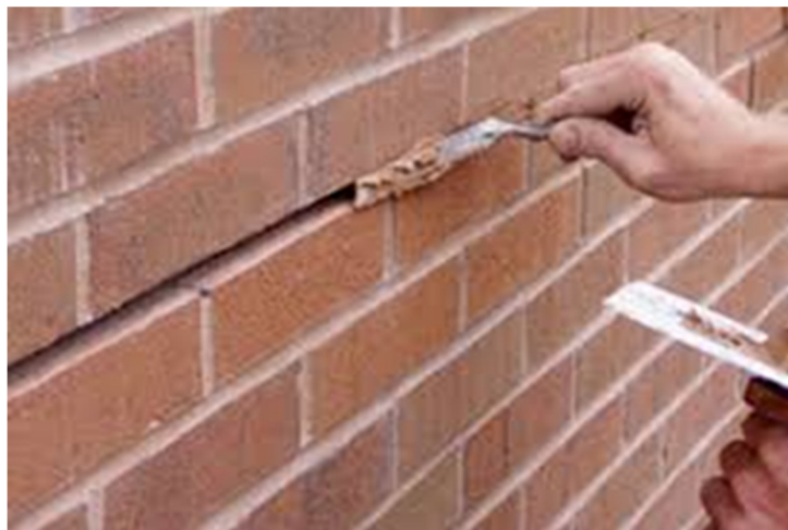
Grinding & Repointing or "Tuck Pointing" Exterior Brick
